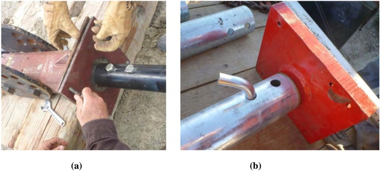
**Figure 8. Foundation attachment unit (a) connected to a 9 cm (3.5") diameter pile (b) attached to the helical pile**
